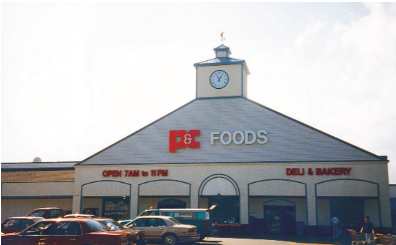
P&C Foods of Canastota, New York is one of thousands of supermarkets nationwide already realizing the significant energy savings that desiccant dehumidification systems offer.
